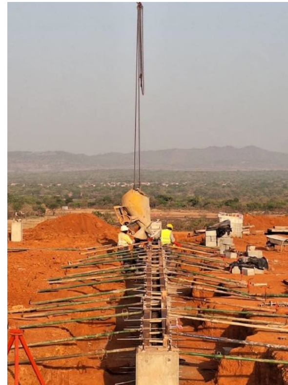
Casting ground beam for plant workshop at Kiniero
