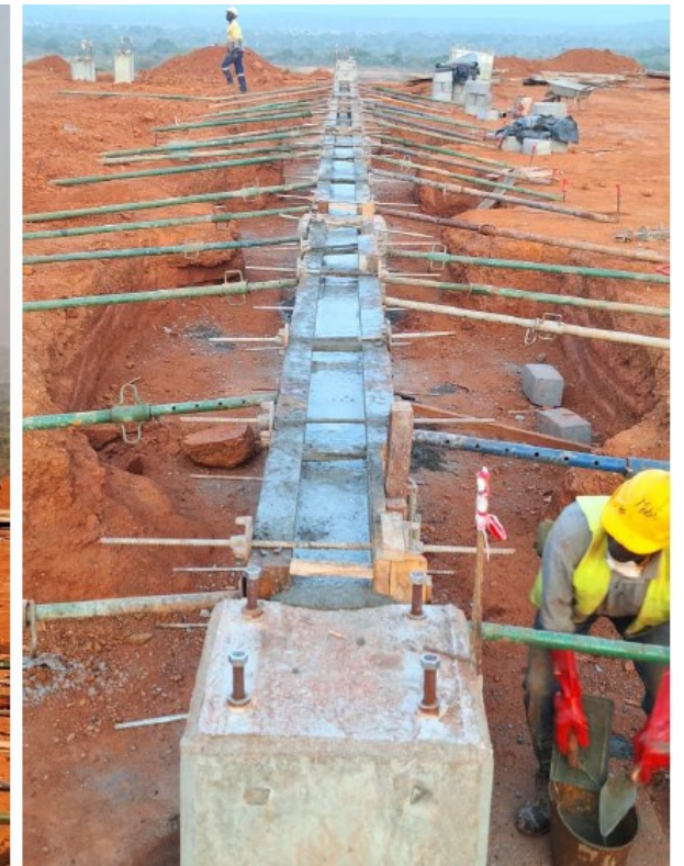
Casting ground beam for plant workshop at Kiniero
