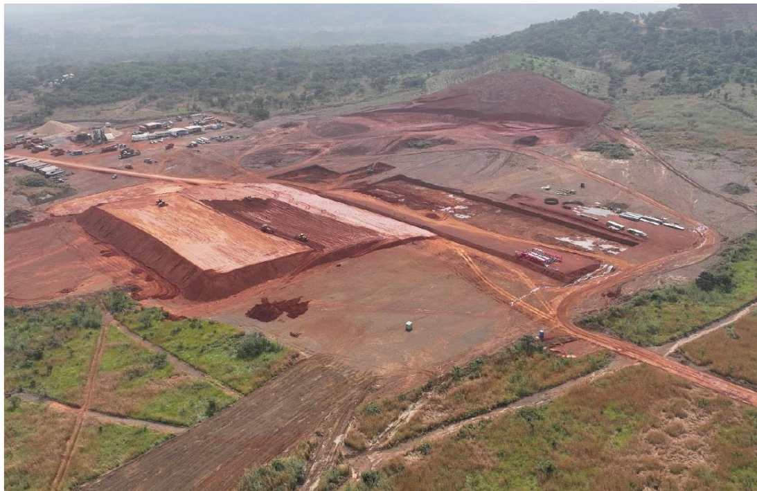
Figure 5: Plant Earthworks construction
