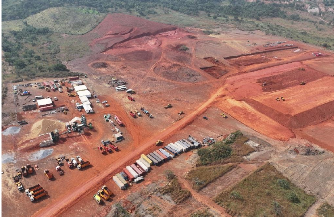
Figure 4: Construction site overview with KCP (Wacom Group) construction area
