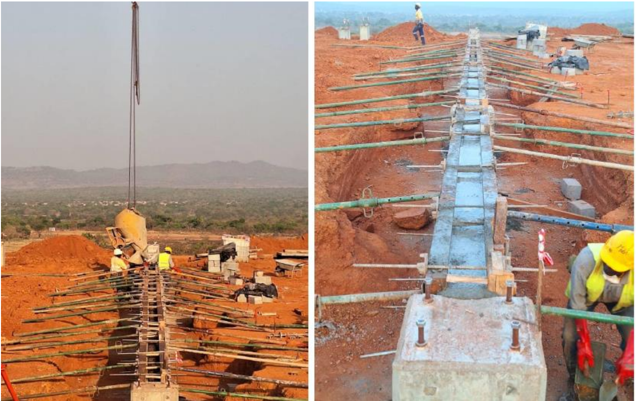
Figure 2 - Casting ground beam for plant workshop at Kiniero
