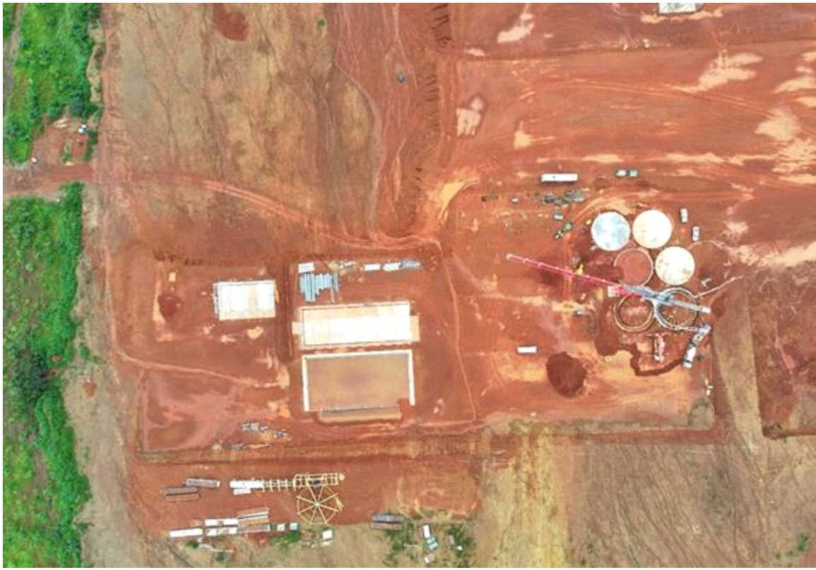
Figure 3: CIL Ring Beams
