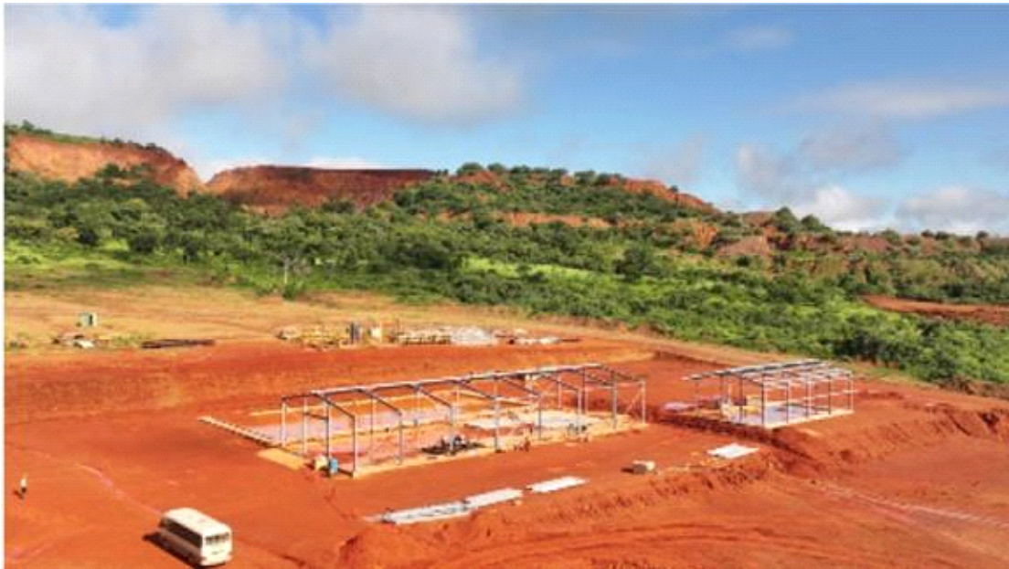
Figure 4: Steel frames for reagent shed
