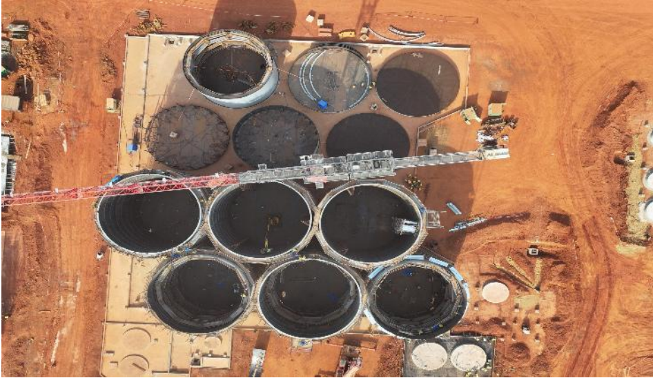
2. Kiniero CIL tank erection top view
