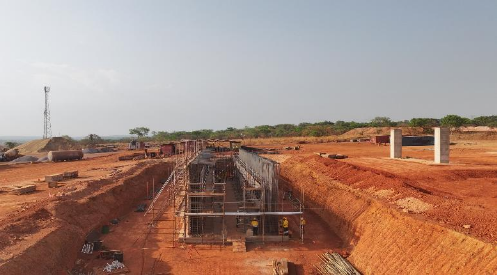
3. Reclaim tunnel concrete structure taking shape.
