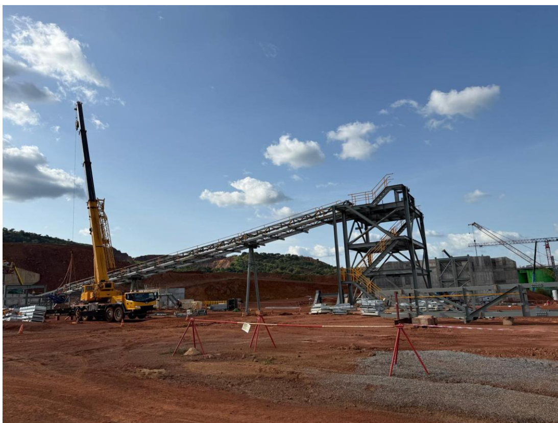
Figure 5: Stockpile feed conveyor truss modules erection (13 October 2025)
