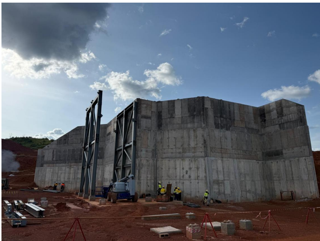
Figure 8: Oxide crushing steel erection progress (13 October 2025)
