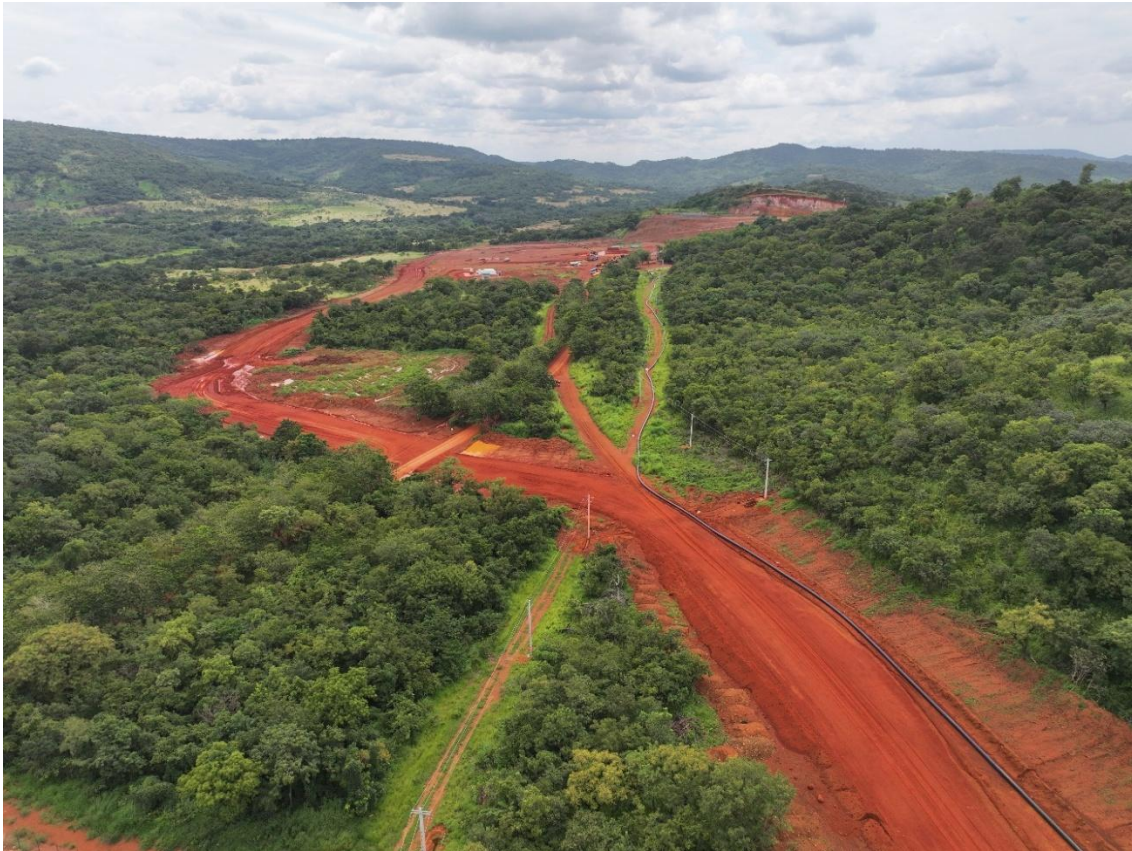
Figure 13: Overland piping installation (12 October 2025)
