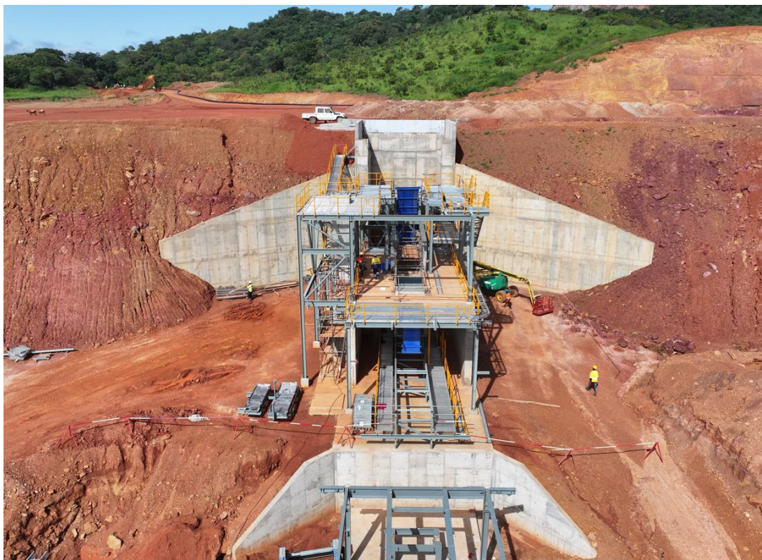
Figure 7: Primary crusher steel erection progress (11 October 2025)
