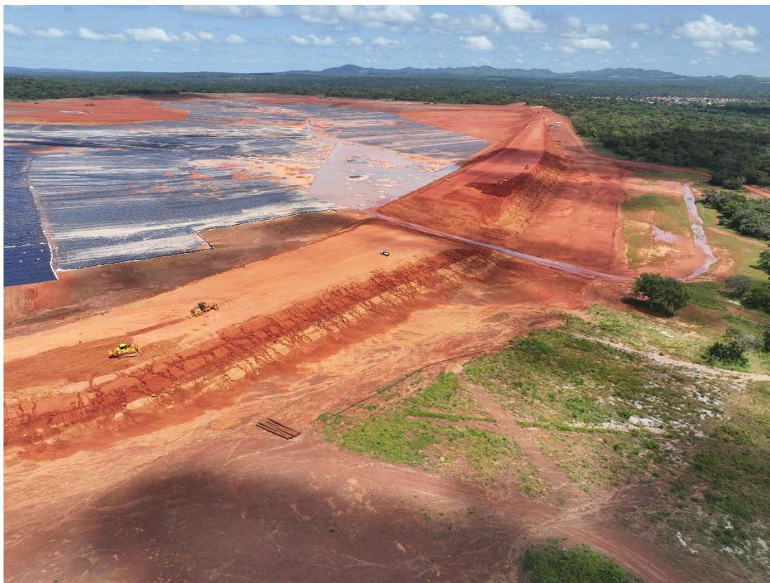
Figure 4: Tailings storage facility showing the extent of lining and main embankment construction (12 October 2025).
