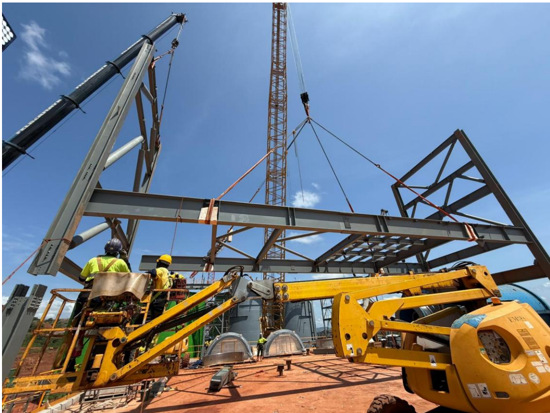
Figure 3: Mill classification tower steelwork lift (13 October 2025)
